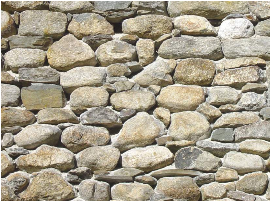
Fig. 25 Detail of interior masonry wythe showing rounded faces and arrises, with looser galleting.
