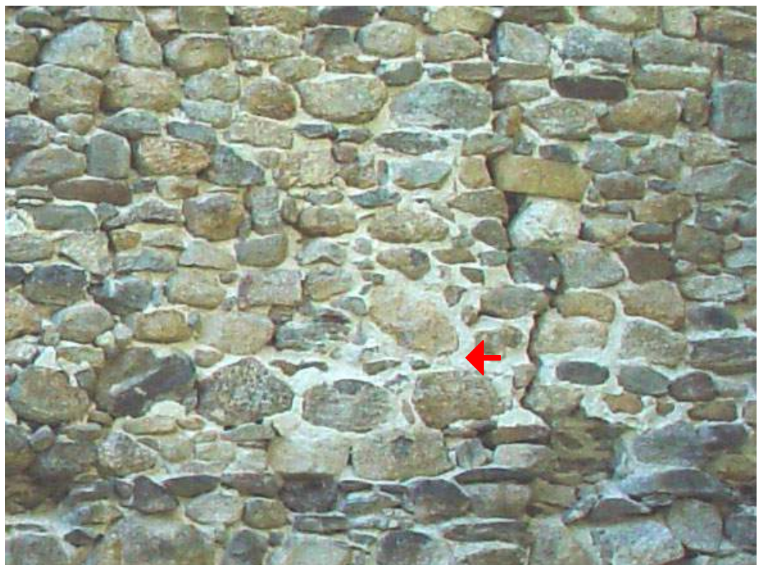
Fig. 29 Pointing repairs executed with incompatible Portland cement mortar.
