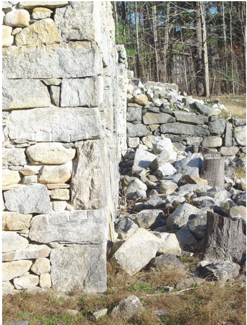
Fig. 29 Pointing repairs executed with incompatible Portland cement mortar.
