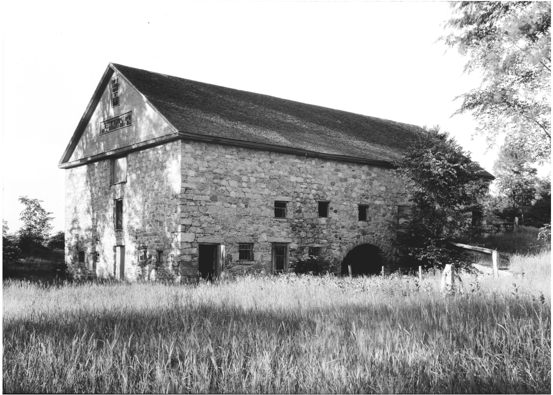
Fig. 16 View from southwest showing beginnings of stone masonry deterioration. (HABS Photograph by Stanley P. Mixon, July 1940)
