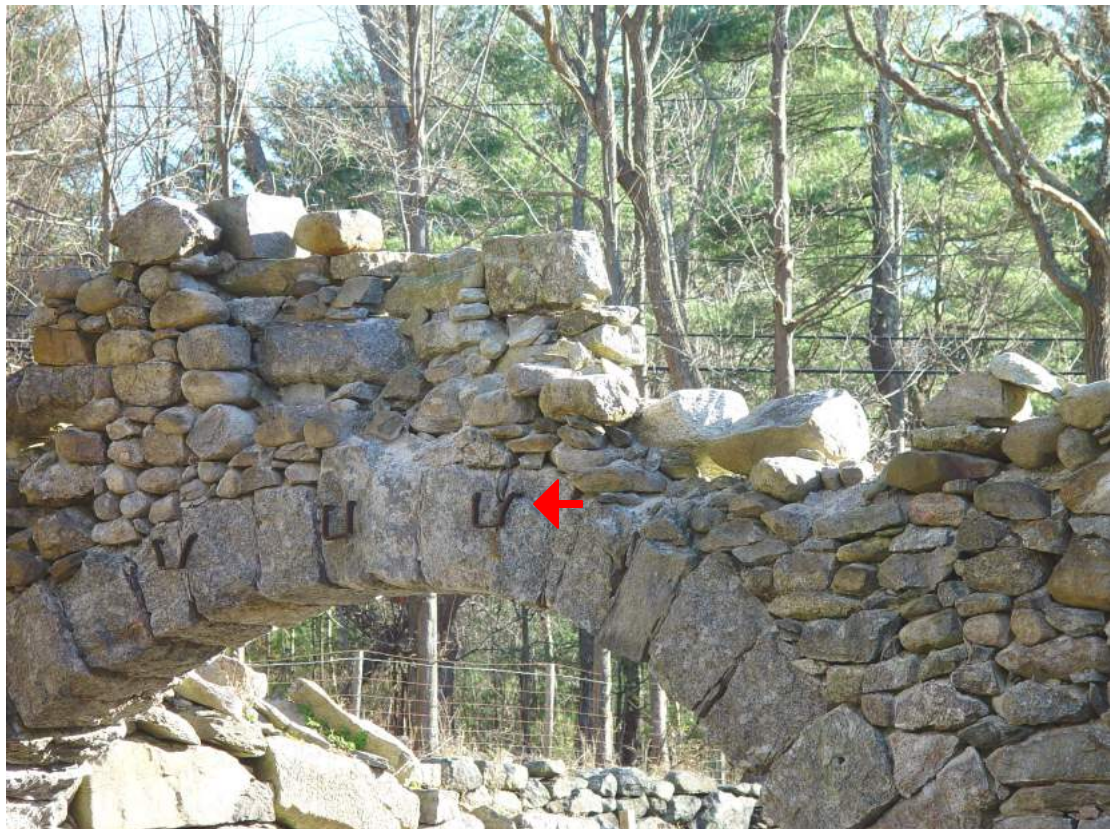
Fig. 11 Iron joist hangers on interior face of south arch.
