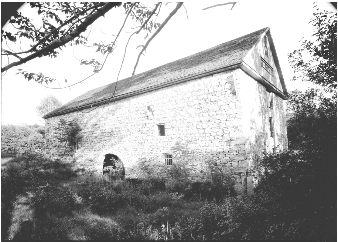
Fig. 13 North elevation showing gutter along eave, and remnant of wood conductor hanging at the northwest corner. (HABS Photograph by Stanley P. Mixon, July 1940)
