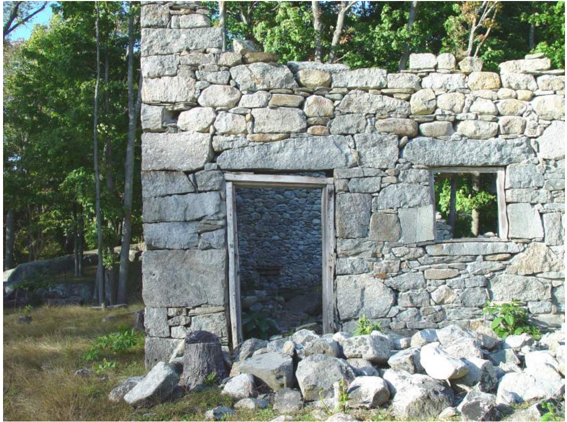
Fig. 2 Dressed exterior granite quoins, jambs, lintels, and sills.
