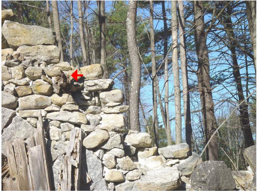
Fig. 8 Interior view of iron framing anchor extending through masonry, with remnant of girt attached.
