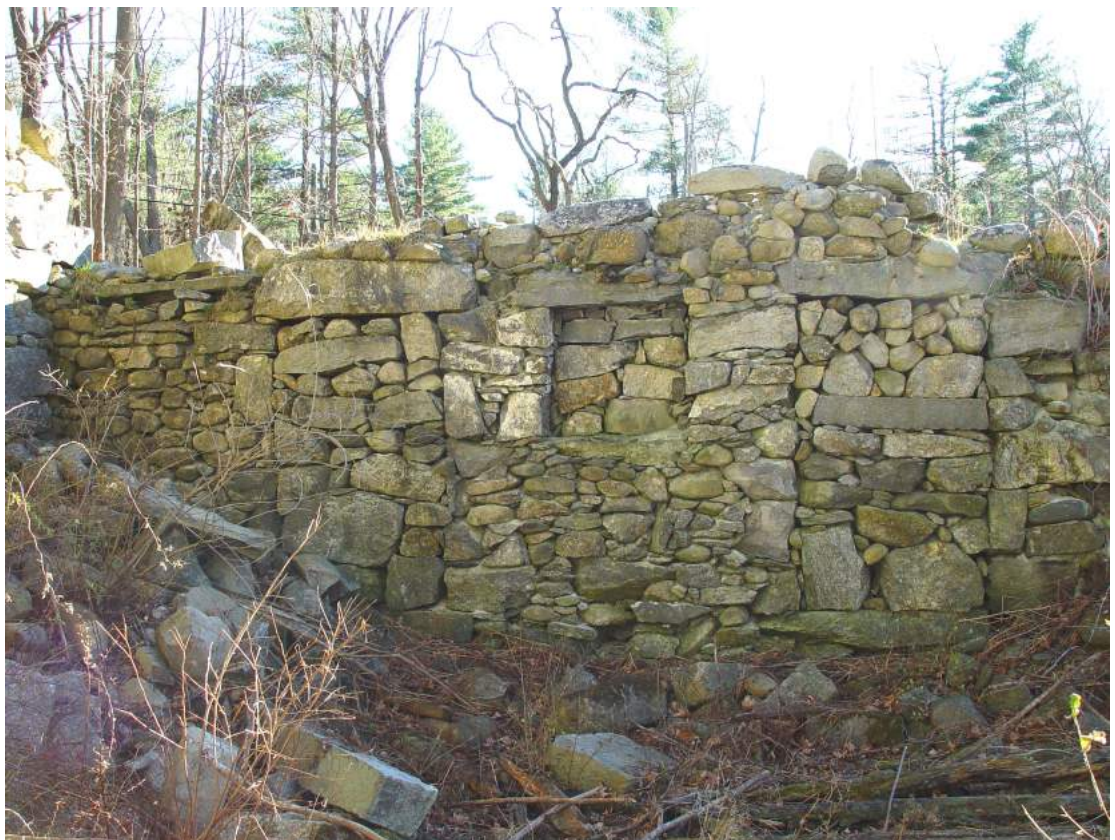
Fig. 5 Altered interior south wall masonry indicating prior window and door openings.
