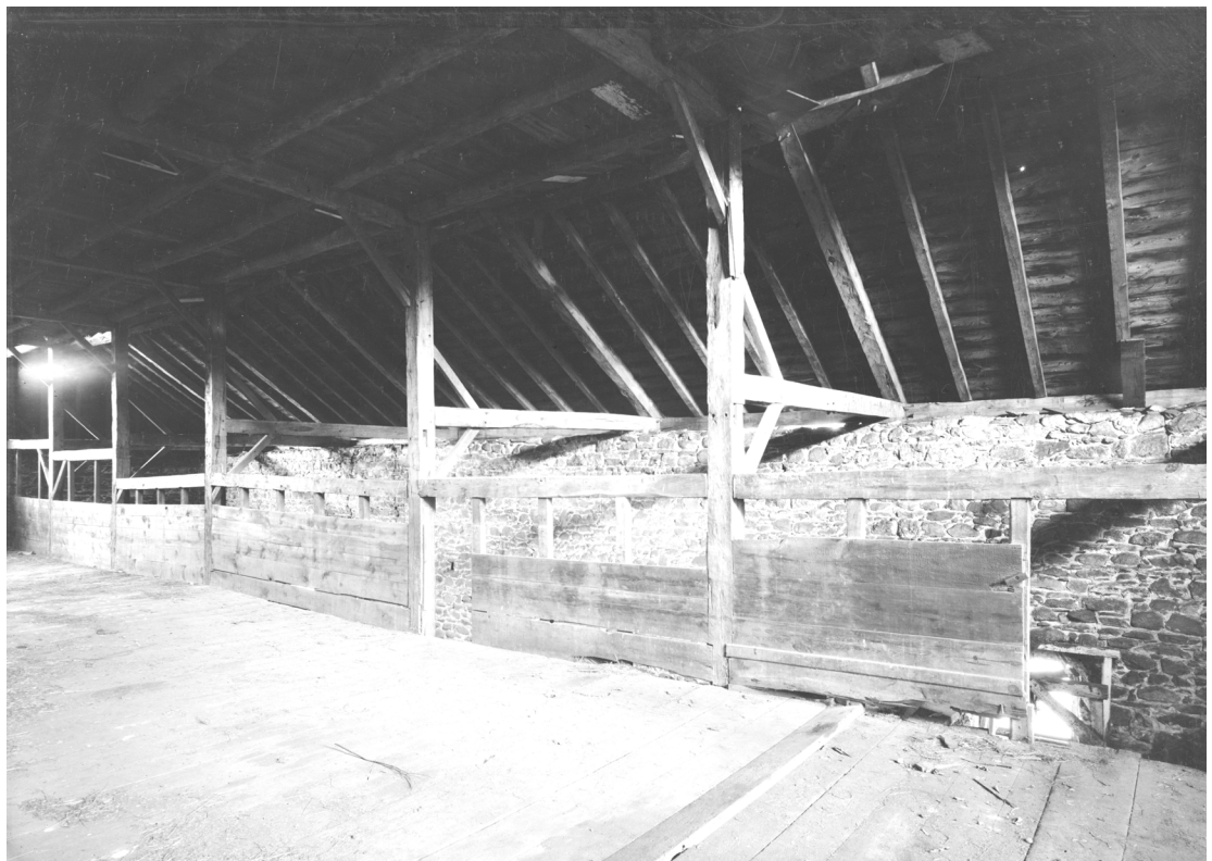
Fig. 7 Interior framing bents with diagonal braces at lateral girts. (HABS Photograph by Stanley P. Mixon, July 1940)
