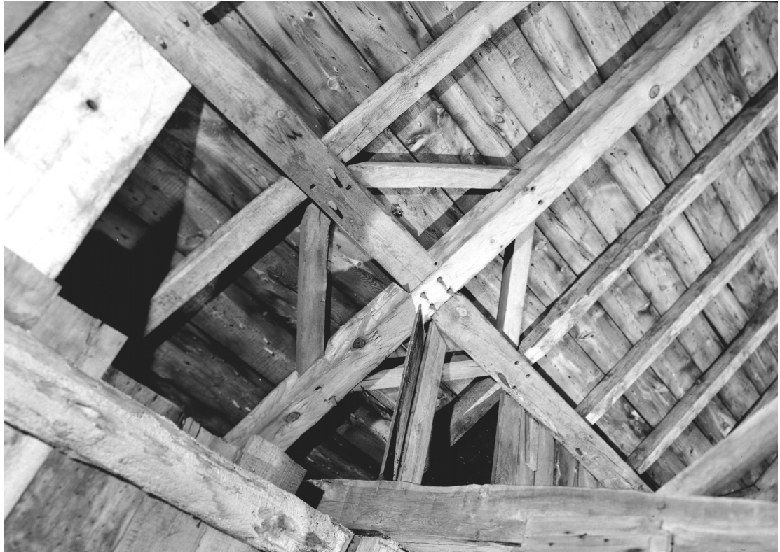
Fig. 12 Roof framing with diagonal braces at intersection of principal rafters and purlins. (HABS Photograph by Jack E. Boucher, August 1963)
