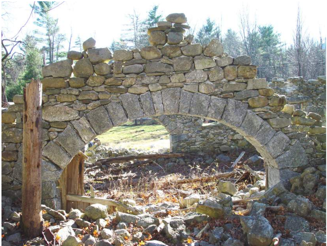
Fig. 33 Exterior of north arch, showing stone faces set flush with plane of wall.
