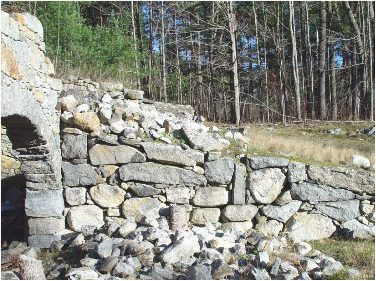
Fig. 35 Dry-laid ramp cheek wall semi-engaged to jamb of south arch.
