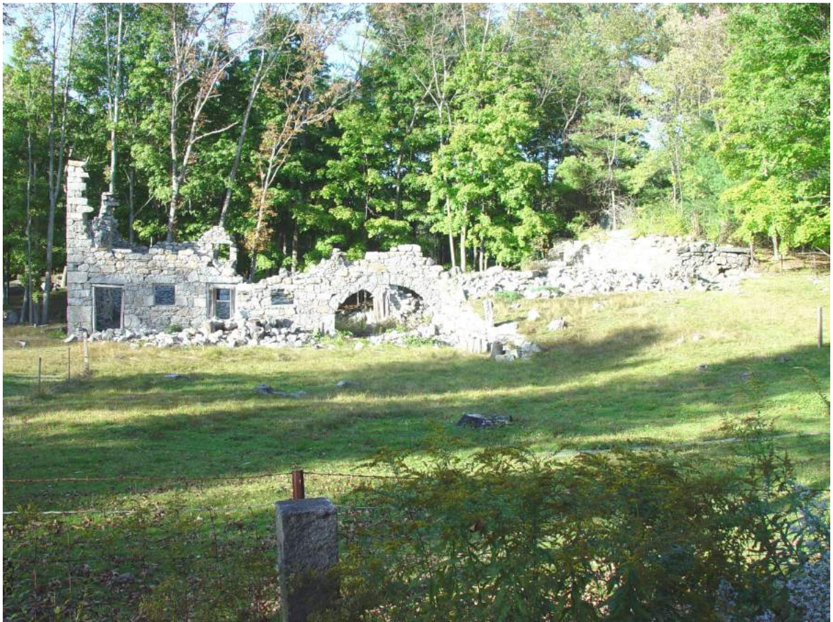
Fig. 1 General view from south.
