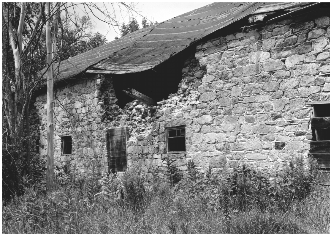
Fig. 21 Breach in south wall stone masonry, east of arch. (HABS Photograph by Jack E. Boucher, August 1963)
