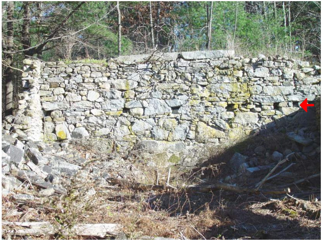
Fig. 10 Joist pockets in east wall interior masonry.
