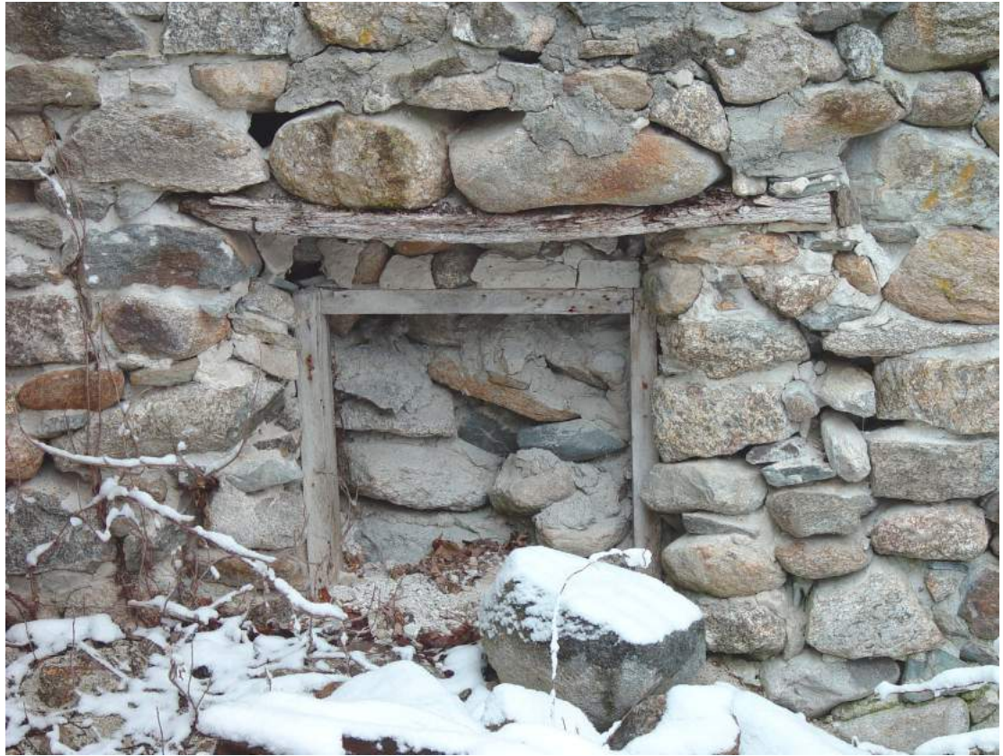
Fig. 6 Abandoned opening at west end interior of north wall, incorporating wood lintels.
