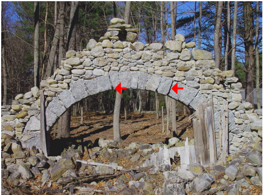
Fig 34 Interior of north arch, showing inconsequential face deviation from the wall plane due to minor variations in stone thickness.
