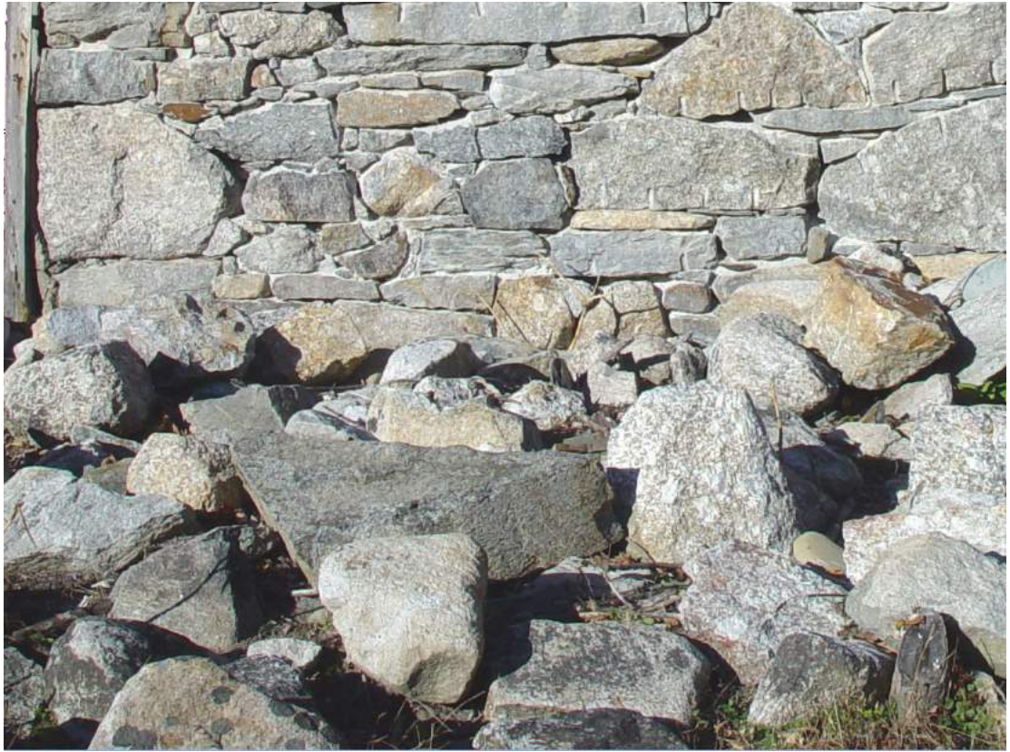
Fig. 24 Detail of exterior masonry wythe showing squared faces and arrises, with tight galleting.
