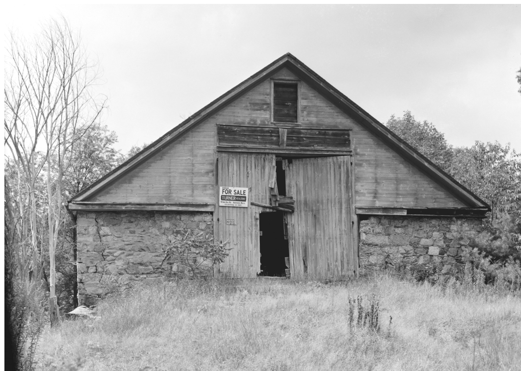
Fig. 15 East elevation showing wood cladding above framed eaves returning across gable. (HABS Photograph by Jack E. Boucher, August 1963)
